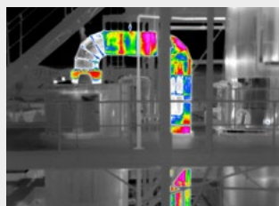
Industrial pipeline inspection
