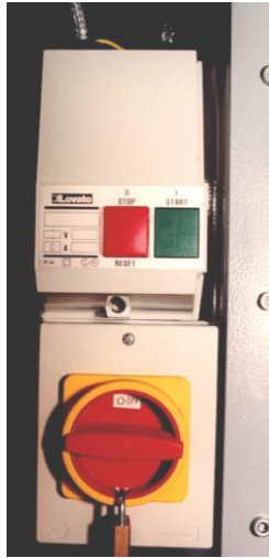
Lockable electrical isolator for added safety
